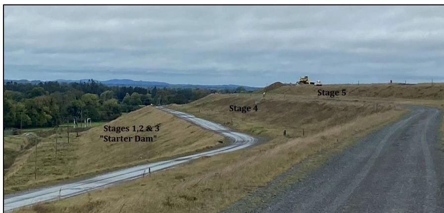
Figure 7: Embankments side profile
